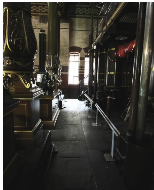
Route to Switch Room
